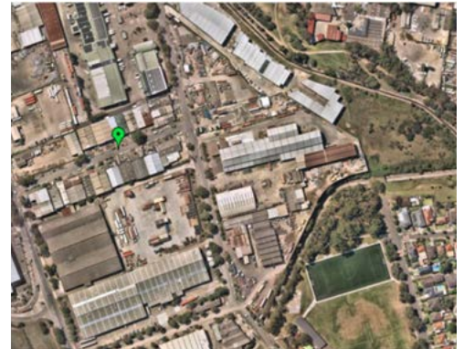
Coxs Creek confluence with Cooks River and South Strathfield Industrial area
